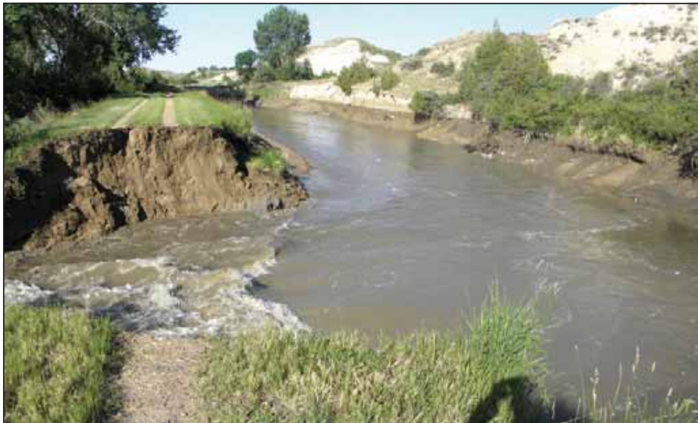
Water pours out of the main canal through the 40 foot washout that occurred south of Savage at the end of June.
