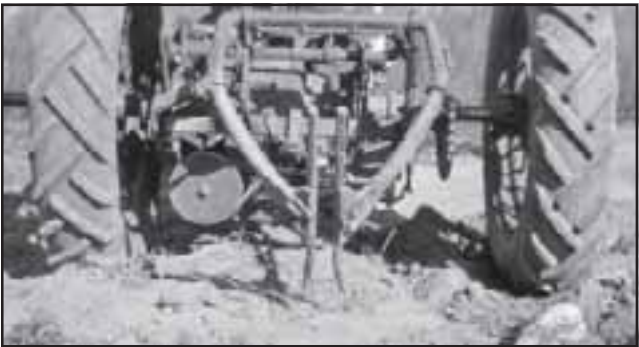
This puller brought the beets to the surface after being topped by the homemade beet topper, 1942.
