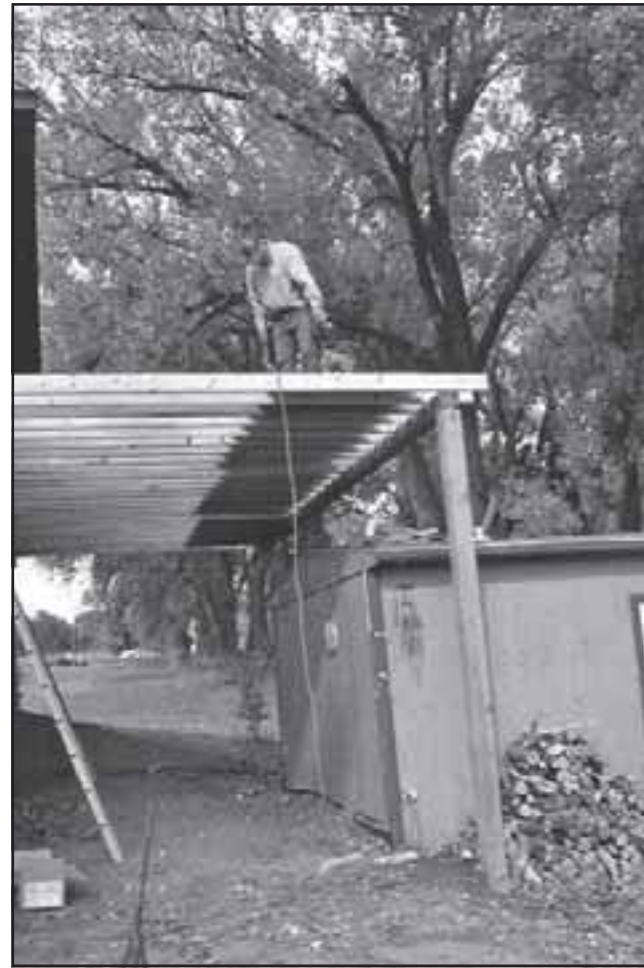
Building the roof.
