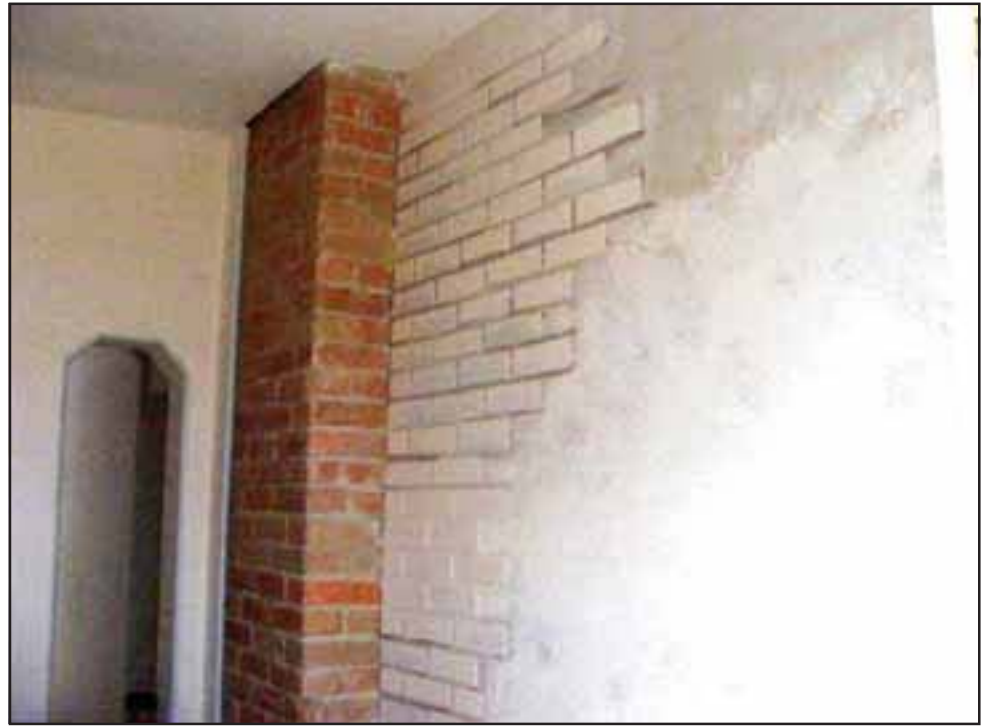
Above: The chimney is real brick, the wall to the right is mud in the Hotel Albert, Fairview.
