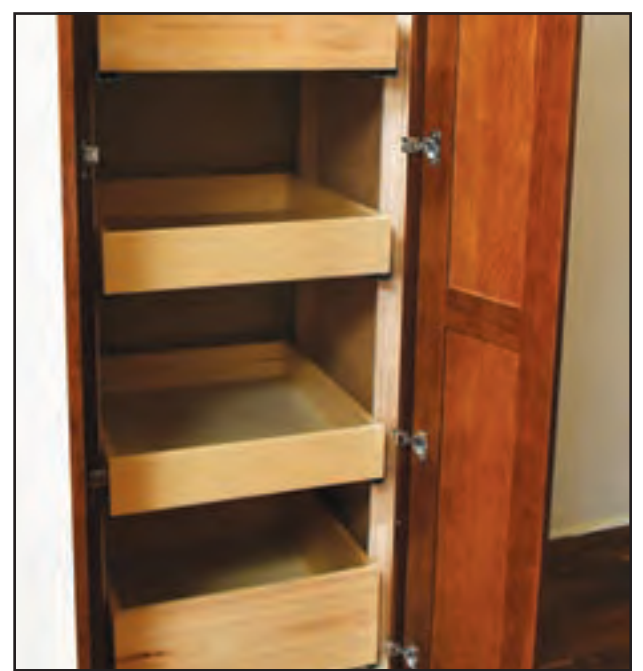
This pantry and the island have many roll out shelves installed for easy access.
