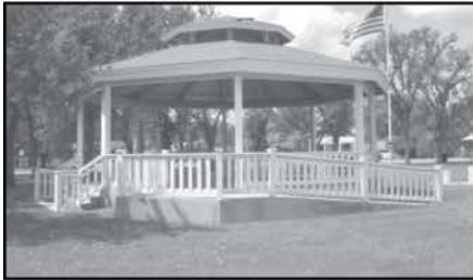
Gazebo in Sharbono Park
