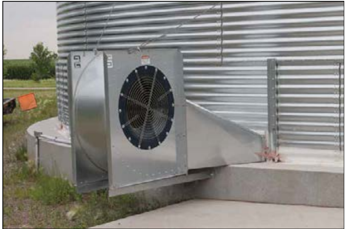
Operating an aeration fan will help move moisture from wet beans to drier beans. (NDSU photo)
